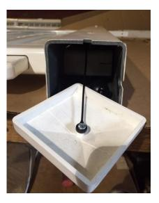
**Step 8**: Place cap on top of post, move the feet into the correct position, connect bungee to adjacent panel if need be, and you are all set!
